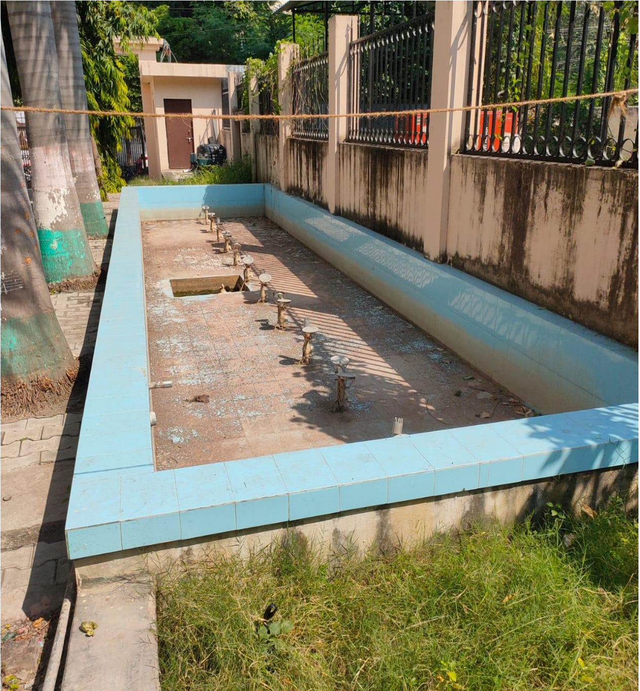
Fountain with water conservation system
